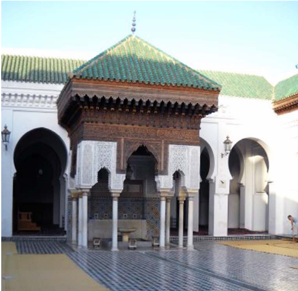
Al-Qarawyyine Mosque in Fes, Morocco
